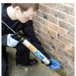
Dryzone's high degree of effectiveness can partly be explained by the fact that it is considerably stronger than competing products (Dryzone contains four times more active ingredient than typical competing DPC injection creams). However, the blend of active ingredients in Dryzone has also been carefully selected to ensure that it is able to spread and cure to form an effective DPC in walls of all types.
